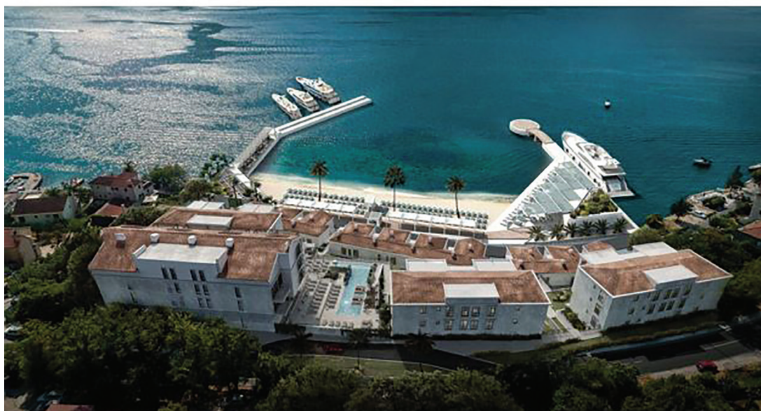
Photograph 6: Location “Camp” after the construction of the complex and the beach filling (taken from the Allure Palazzi Kotor Bay website)
